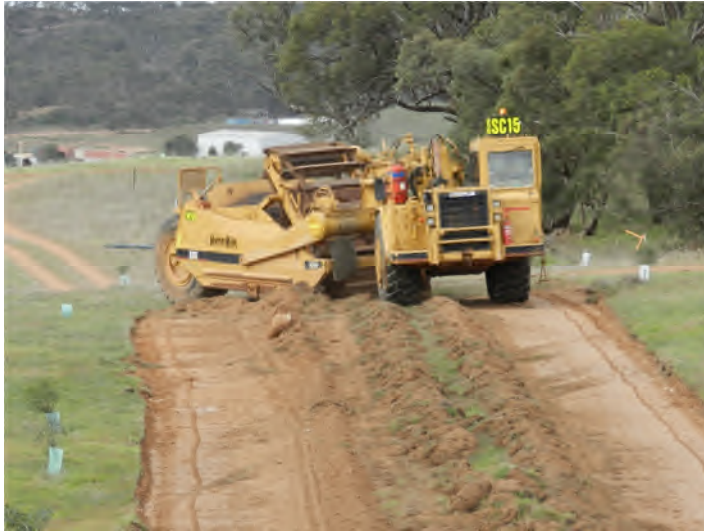
Figure 27: Lifting windrowed topsoil from sowing bays with a Cat Scraper (NW Woodlands), April 2013
