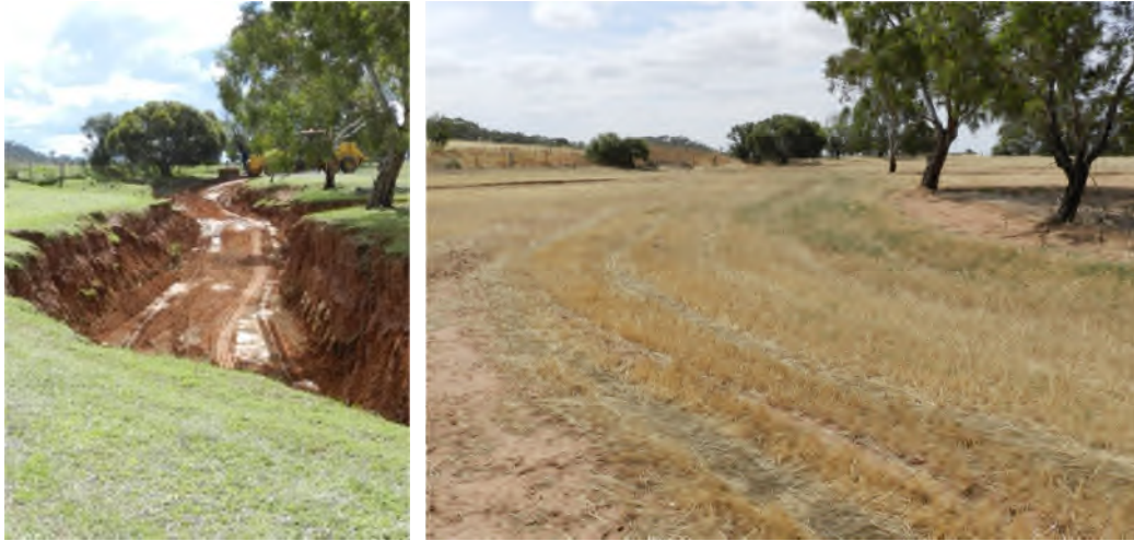
Figure 29: ‘Before and after’ photos of Stage 1 gully erosion backfill completion – Mine Rd. Note that the 3m deep erosion gully has been replaced with a broad, gently inclined grassed waterway with good erosion resistance
