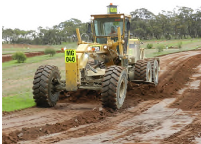
Figure 26: Windrowing topsoil in the middle of sowing bays with Cat grader (NW Woodlands – Kanmantoo Copper Mine)
