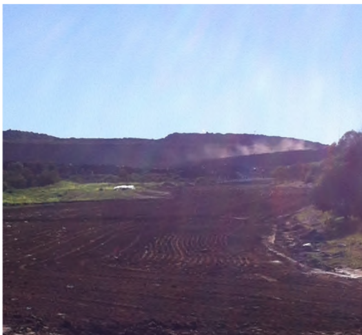
Figure 43: Rehabilitation of Smelter Rd just prior to direct seeding, April 2012. Smelter Rd provides an analogue site for the Mine Rd plantings. It provides a benchmark to track the development of direct-seeded vegetation using the topsoil pre-strip technique.
