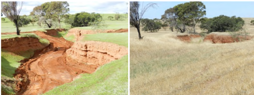
Figure 28: Stage 1 of progressively filling gully erosion with stripped topsoil and creating an improved drainage channel 'before and after' (Mine Rd SEB-Offset areas)
