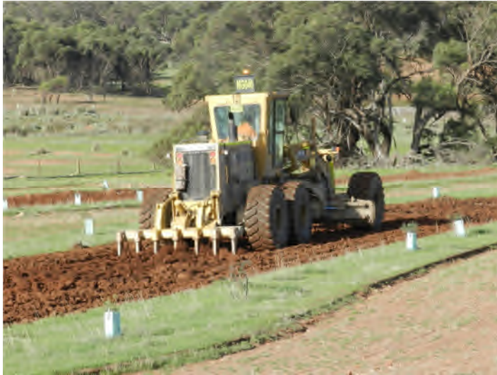
Figure 30: Deep-ripping with grader to improve water infiltration prior to initial cultivation with power rake (NW Woodlands – Kanmantoo Copper Mine)
